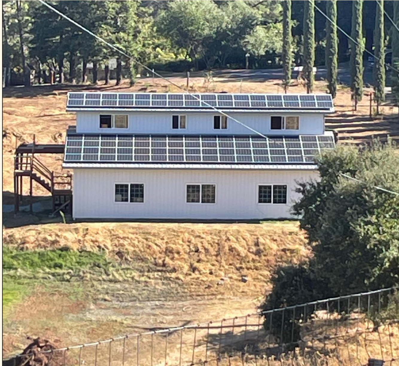
Solar Panel Installed
